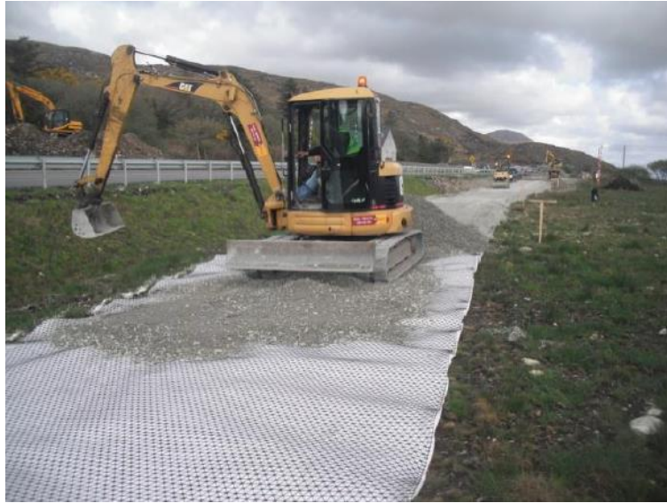
Figure C.4 Geotextile reinforced unbound granular layer construction
