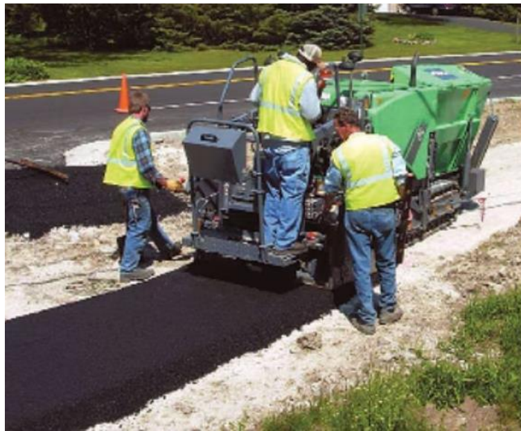
Figure C.1 Narrow width bituminous material paver
