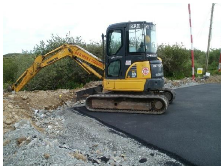
Figure C.3 Lightweight backacter for cycleway construction
