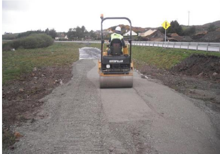
Figure C.2 Lightweight roller compactor equipment for cycleway construction
